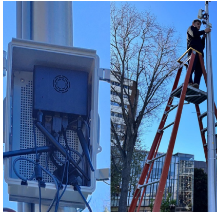
Sensor installing on site
