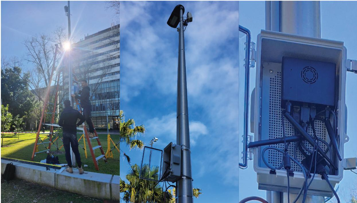
To support this sensor kit, you will need at least one power source to supply power to three devices: a GoPro, an Nvidia Jetson, and a mobile hotspot router. It is crucial that the mobile hotspot router includes an Ethernet port; without this, the connection between the GoPro and Nvidia Jetson may become unstable. We highly recommend using a hotspot router with an Ethernet port for this set-up. In this project, we used a device recommended by a local provider.
